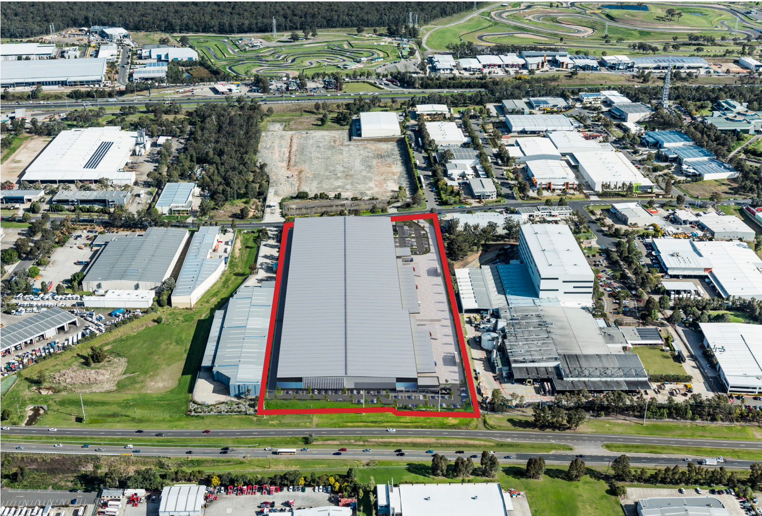
AERIAL IMAGE OF PROPOSED DEVELOPMENT LOOKING SOUTH
